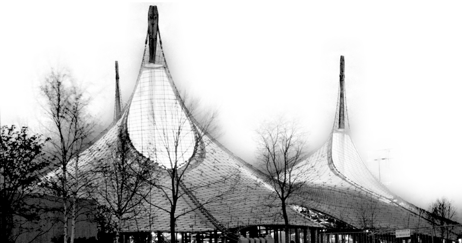
Figure 9: Frei Otto & Rolf Gutbrod, German Pavilion, Expo 1967 (Otto, 1967) The first large cable net structure with fabric cladding
